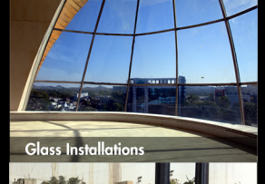
Membrane and Glass Roofs
